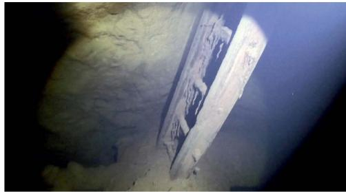
Above: 'Rusticle'-type protrusions on the rungs of a submerged ladder 25m down at the base of a flooded shaft.
